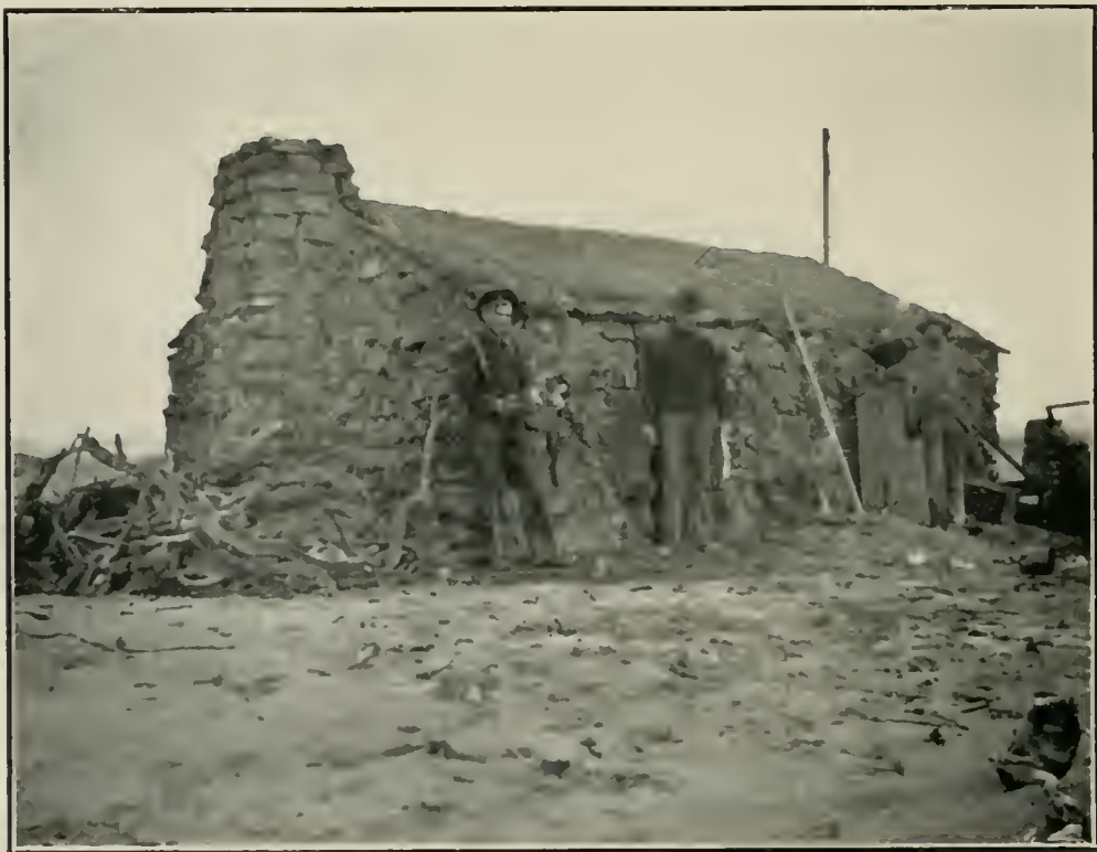
HOUSE OF ROCK SALT, DANBY LAKE, SAN BERNARDINO COUNTY.
